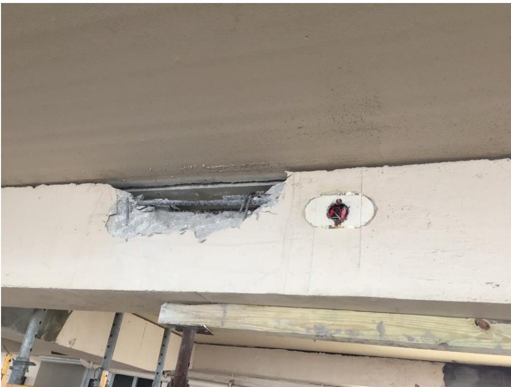
Picture 2: In-progress concrete demolition
