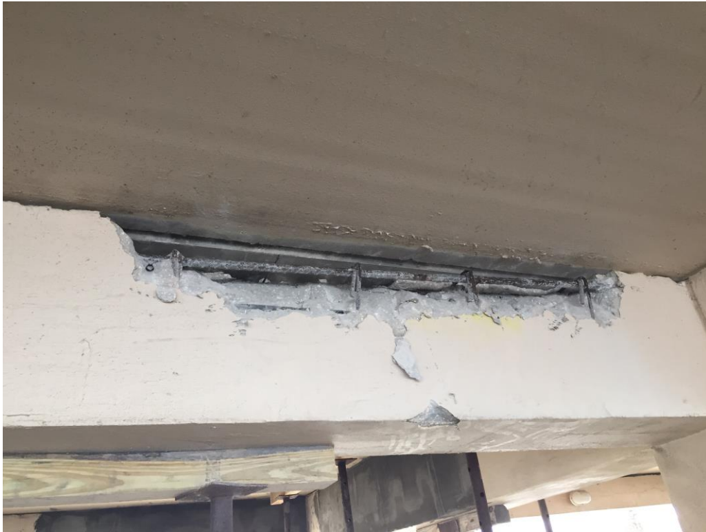
Picture 1: In-progress concrete demolition
